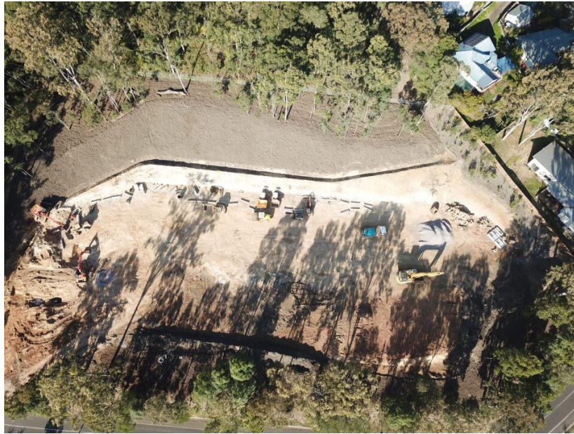
Site ready for handover to the builder
