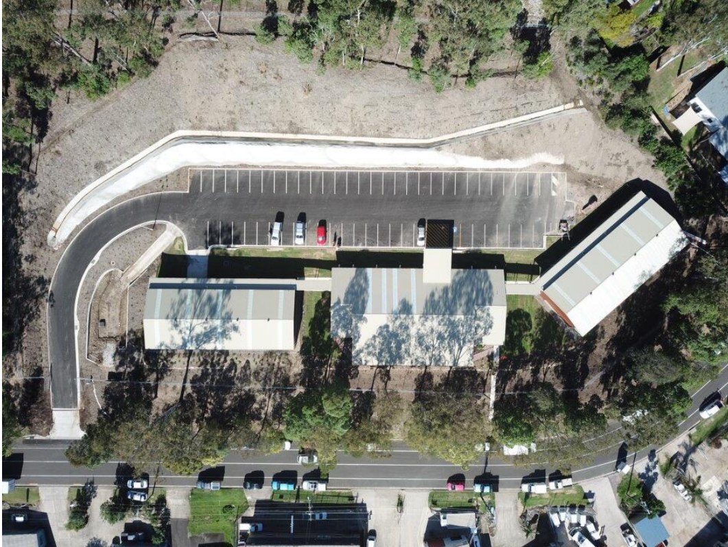
Just after hand over we now had full access
