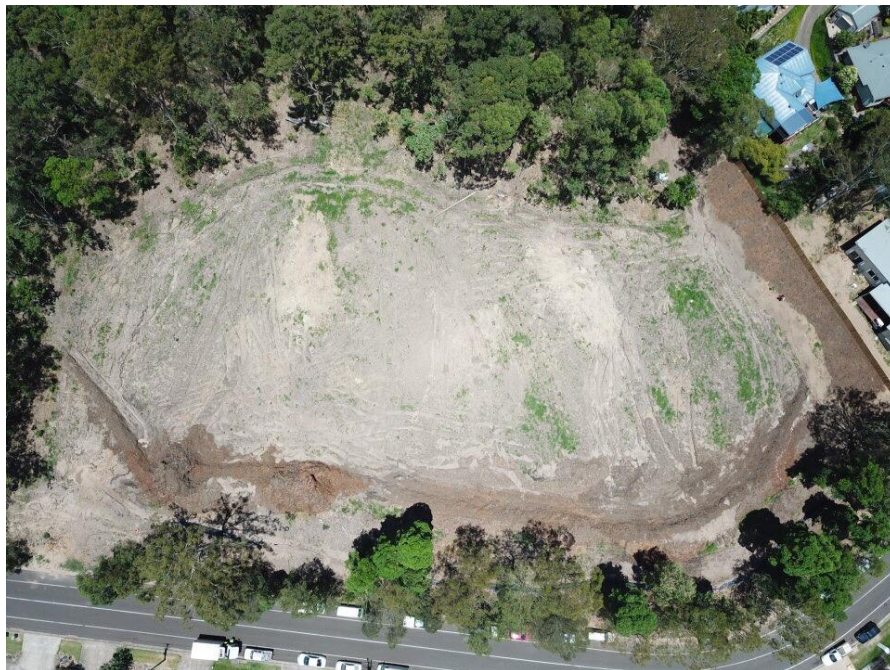
Site cleared and ready to go
