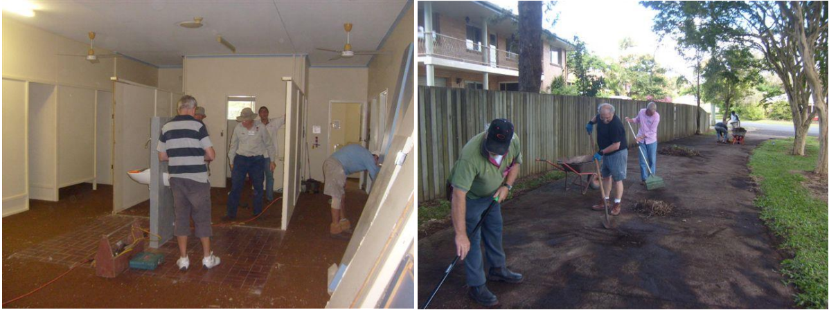
Preparing the site for occupancy – inside and out
